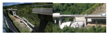
Fig. 4. Pictures showing the section of the Castro viaduct in the province of Leon has collapsed during refurbishment work.
