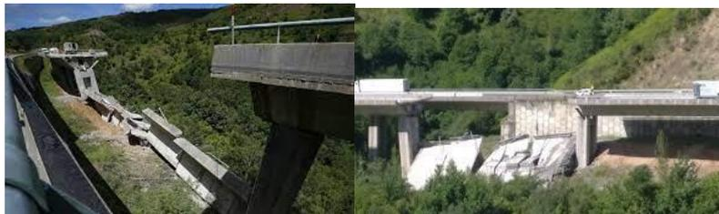
*Fig. 4. Pictures showing the section of the Castro viaduct in the province of Leon has collapsed during refurbishment work.*
